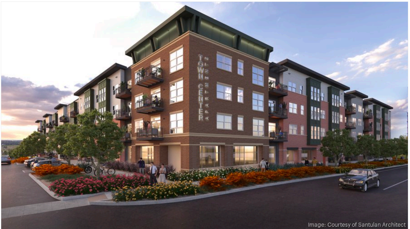
Image: Courtesy of Santulan Architect
